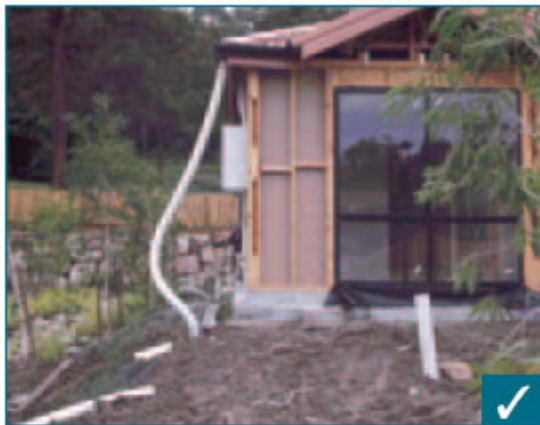
Temporary roof water connection
