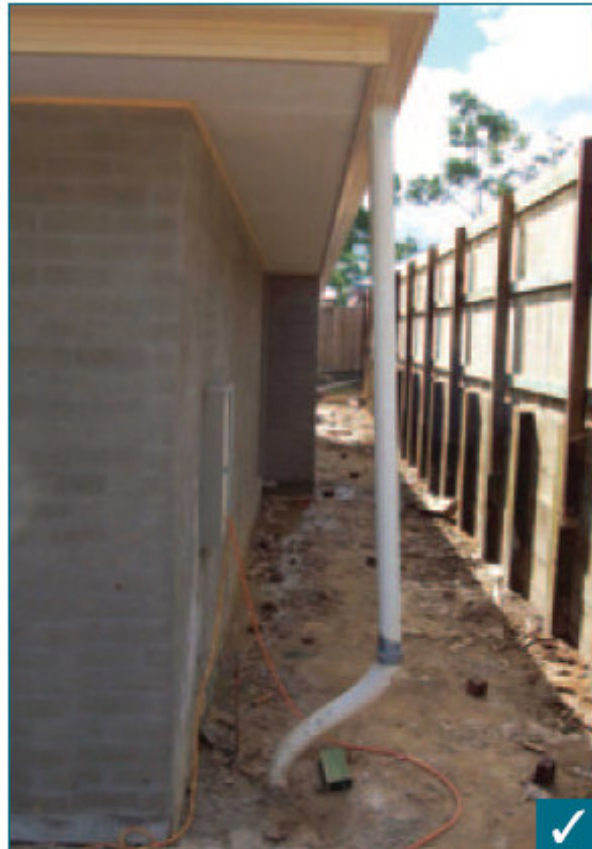
Temporary roof water connection
